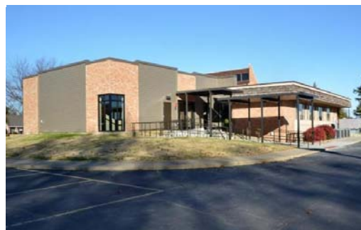
St. Luke Union Church, Bloomington completed building project making the building more accessible.
